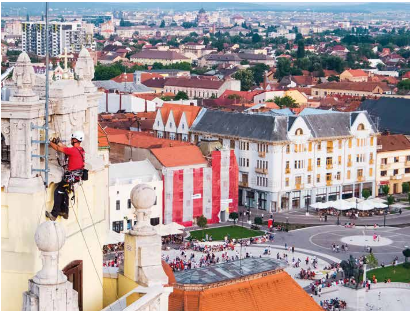
Rope access work on the city hall tower of Oradea.
