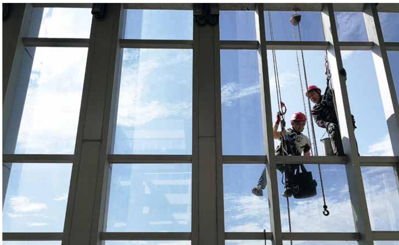
Glass window installation on a skyscraper in Beijing. Instalaciones de cristales sobre un rascacielos. Beijing, China (courtesy of Beijing Speed-Nimble Aerial Protective Equipment Co. Ltd.).
