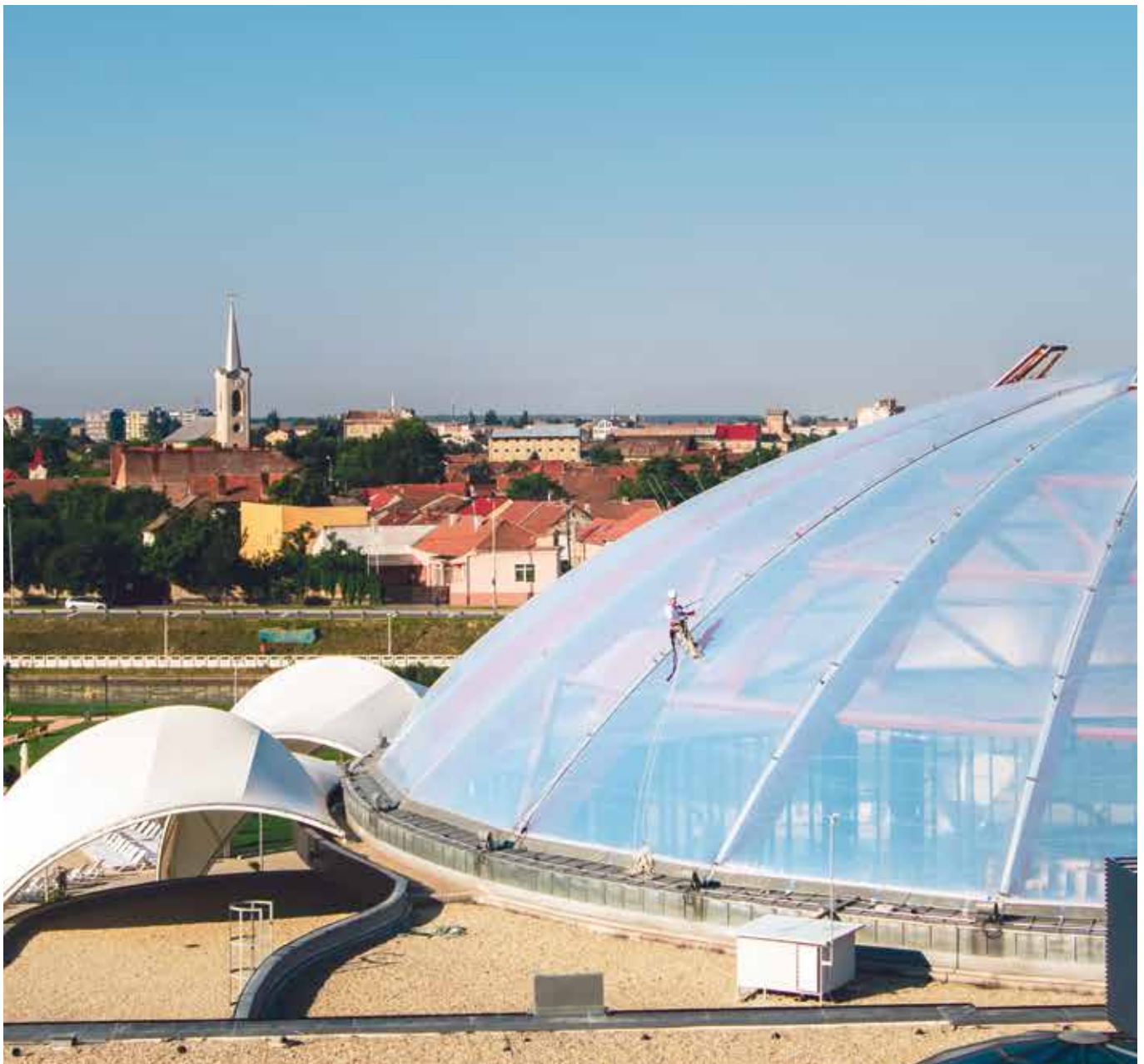
Experiencing the features of the Giant descender on the cupola of the Aquapark Nymphaea. Bajada con el descensor Giant encima de la cúpula del Aquapark Nymphaea. Oradea, Romania (courtesy of Camp Technical Solutions, ph. Amazing Visuals Studio).
